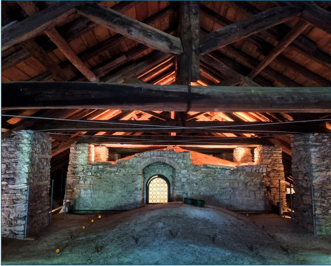
Figure 6. Feltre, Sanctuary of Saints Vittore and Corona, detail of the attic spaces above the central nave. (Source: A. Passuello)
