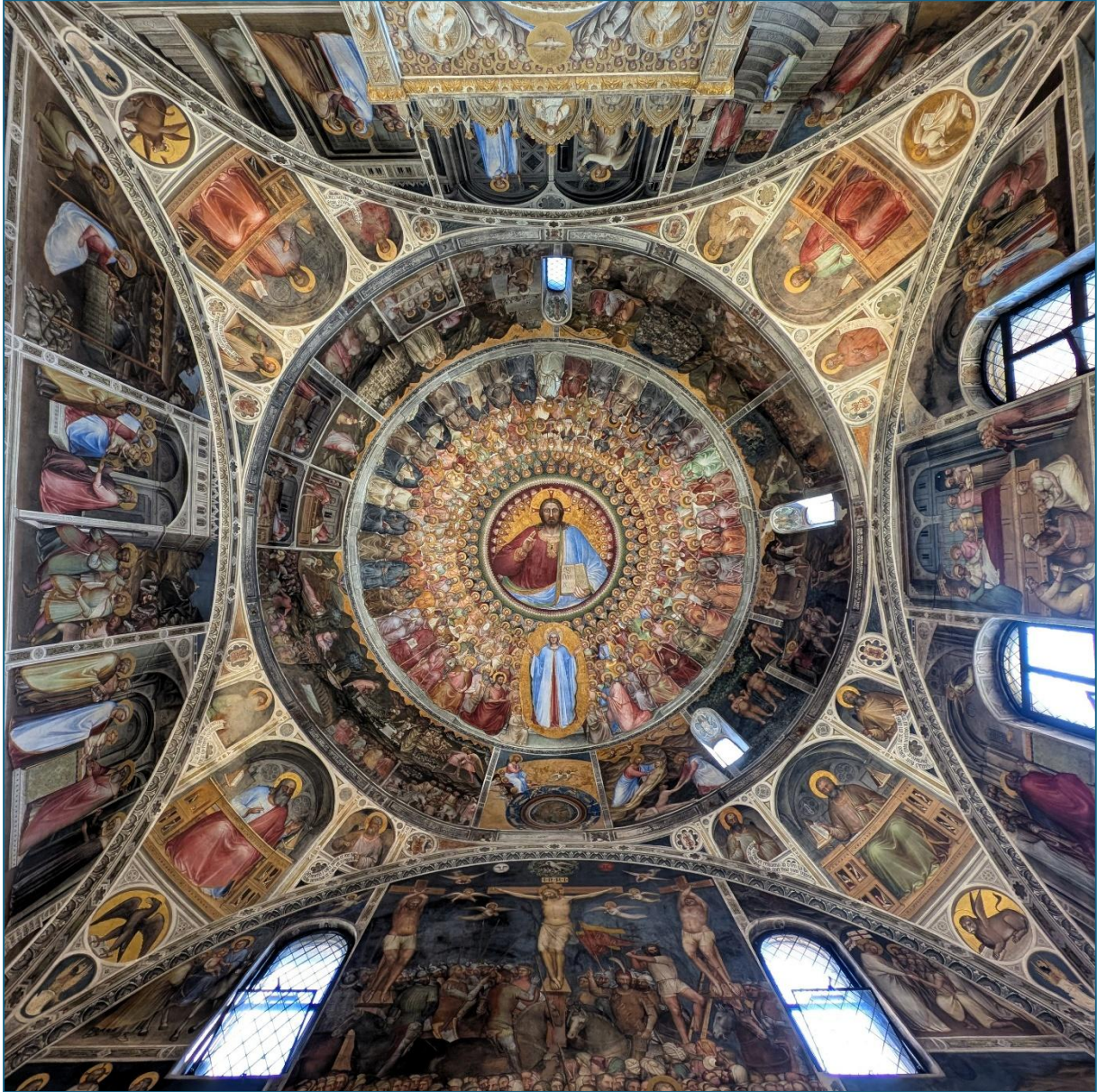
Figure 3. Padua, Baptistery, roofing system with dome and pendentives. (Source: A. Passuello)
