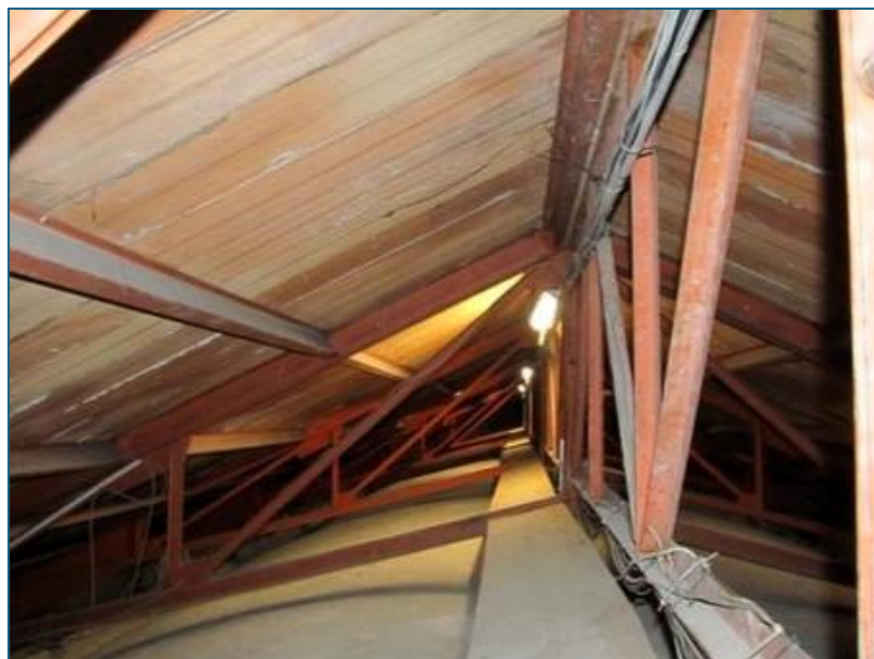
Figure 6. Padua, Scrovegni Chapel, detail of the attic spaces with metal trusses. (Source: University of Padua Thesis Repository )
