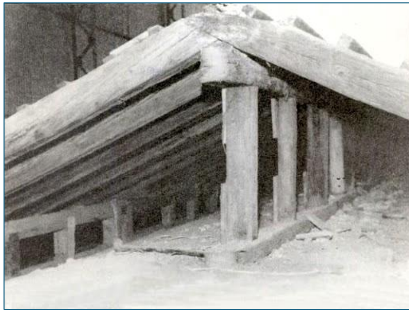
Figure 5. Padua, Scrovegni Chapel, timber trusses prior to the restoration campaigns of the 1960s. (Source: Colabich, Prosdociami & Saccomani, 1964)
