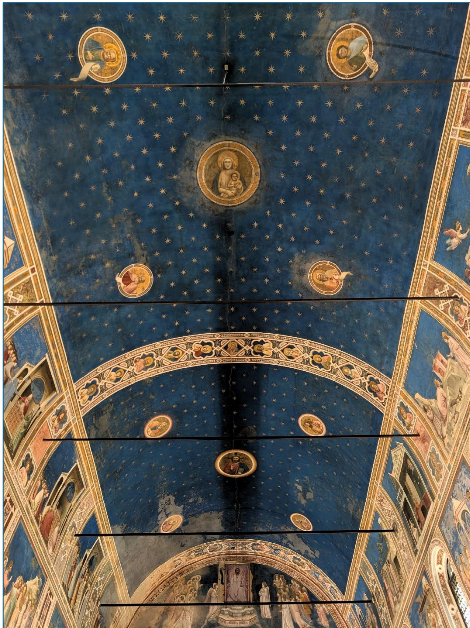
Figure 4. Padua, Scrovegni Chapel, barrel vault. (Source: A. Passuello)
