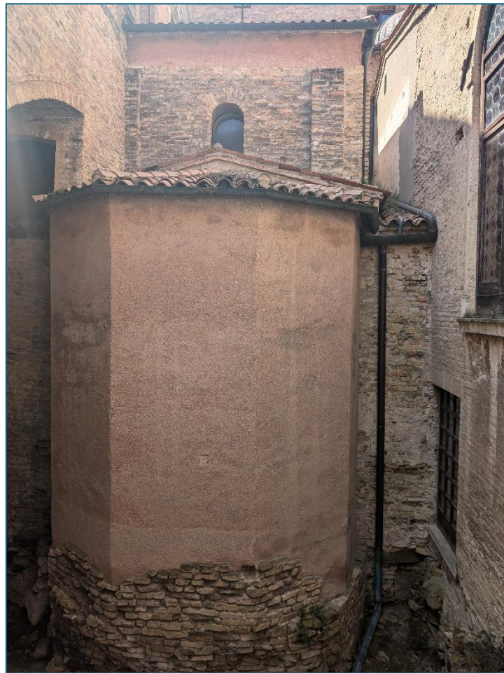
Figure 1. Padua, Church of San Prosdocimo, exterior view. (Source: A. Passuello)
