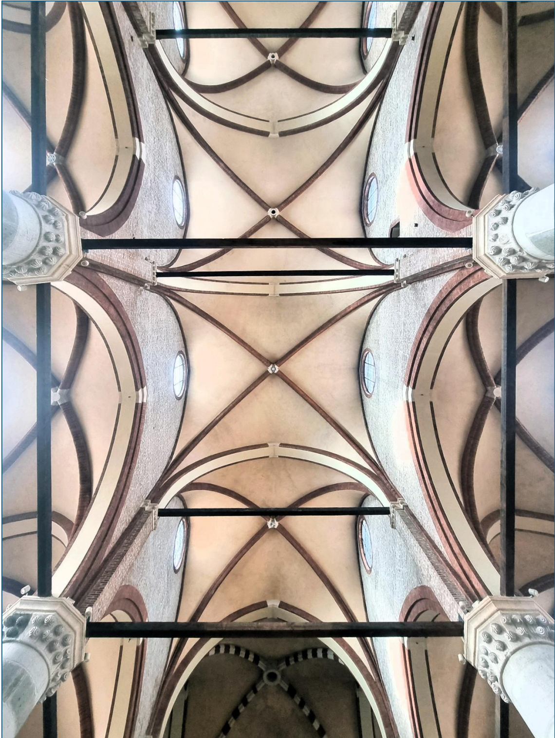
Figure 4. Vicenza, Basilica of San Lorenzo, quadripartite rib vaults of the central nave. (Source: A. Passuello)
