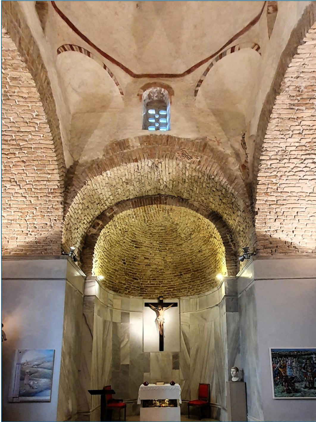
Figure 2. Vicenza, Church of Santa Maria Mater Domini, interior view. (Source: A. Passuello)
