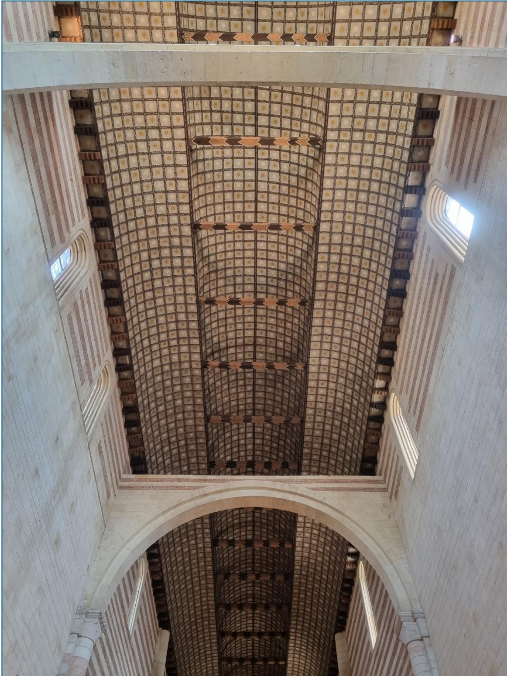
Figure 4. Verona, Basilica of San Zeno Maggiore, inverted ship-hull timber ceiling. (Source: A. Passuello)
